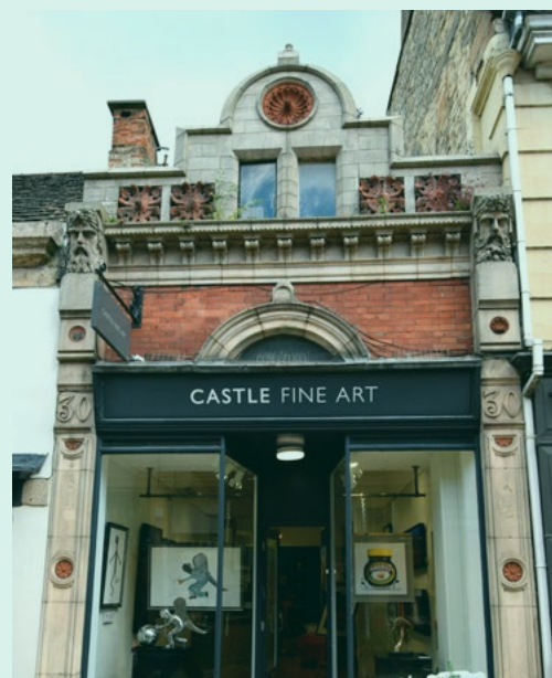
This highly decorative shopfront breaks the mould in Stamford with limestone, timber, brick and terracotta elements.
