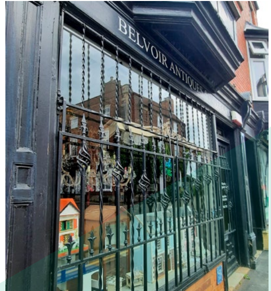
Removable grilles allow customers to see shop displays even when the business is closed. Permanent fixing points are discrete and do not detract from the shopfront.
